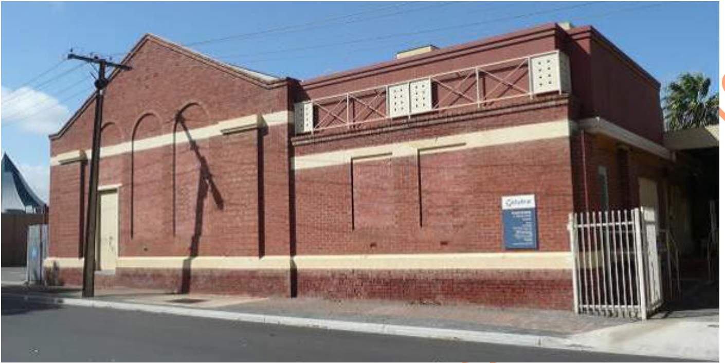
Telephone Exchange, Prospect. Photo source: Prospect Heritage Review, McDougall and Vines
