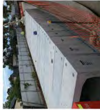
Culvert installation
