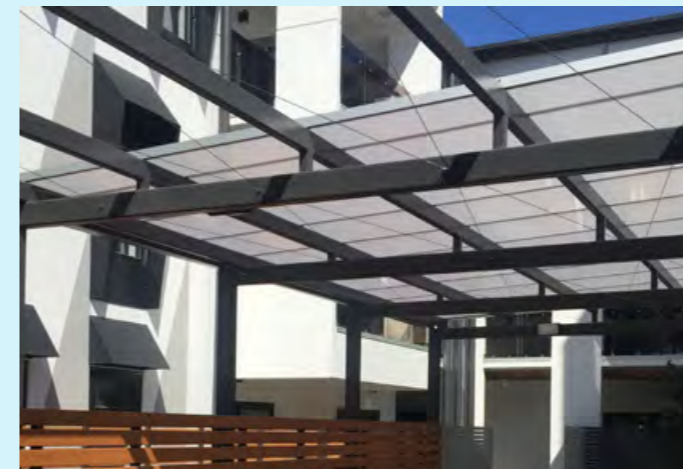
3 Shade structure - solid roof
