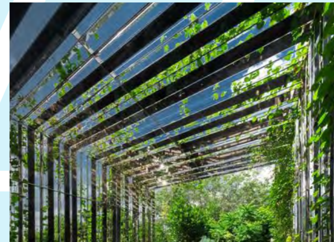
3 11 Permeable trellis roof or screening
