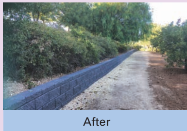
Penfold Park retaining wall - replaced ageing planks with 50m of charcoal blocks. ($15k)
