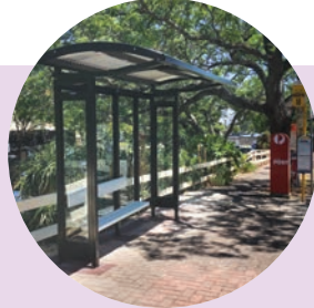
New bus shelter Devereux Rd, Linden Park (Stop 18). ($57k)
