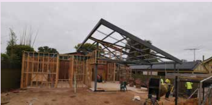
Construction underway on the Dulwich Community Centre
