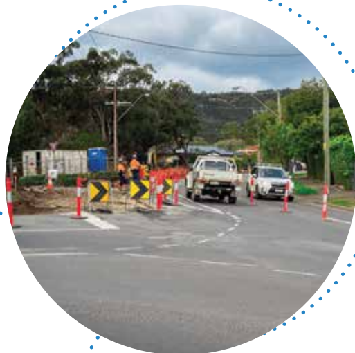
Greenhill Road and Hallett Road intersection works
