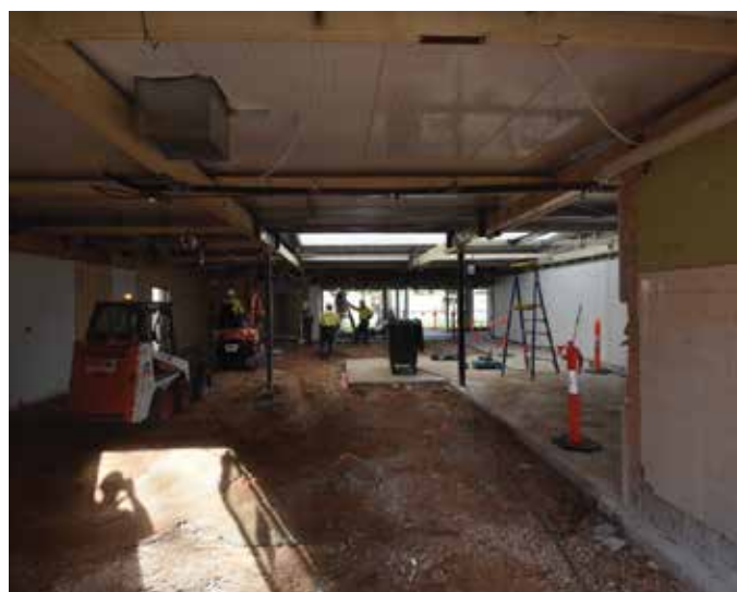
Works are underway at George Bolton Swimming Centre
