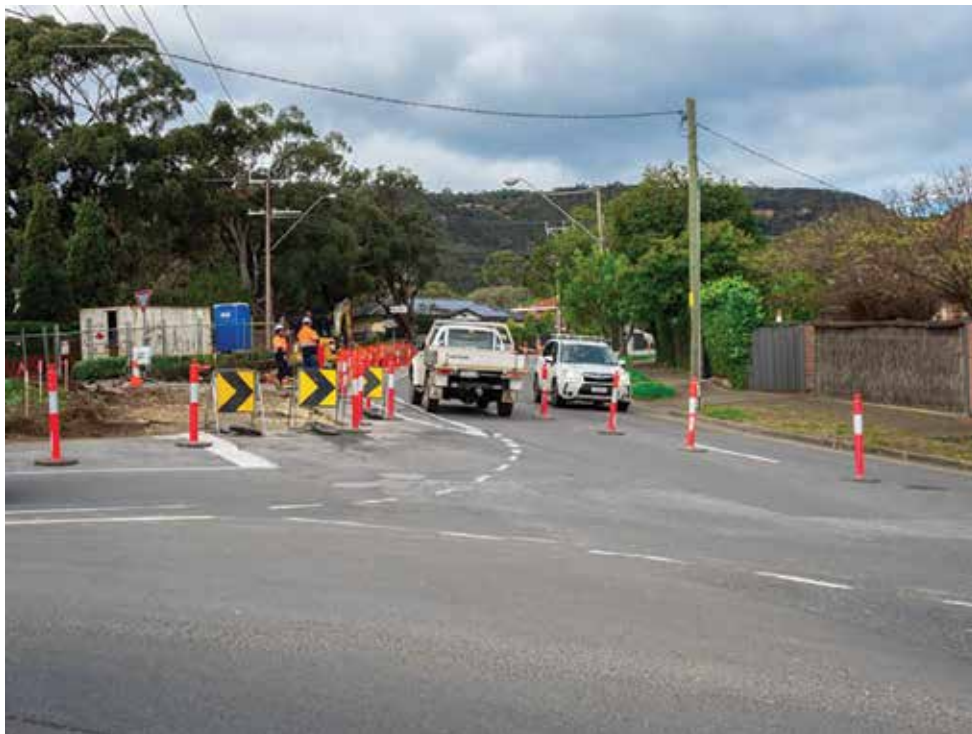
Greenhill Road and Hallett Road intersection works
