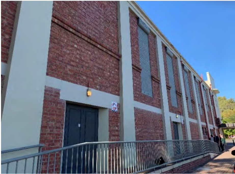
Figure 7: West elevation – note expressed concrete piers (GGA, 2019)
