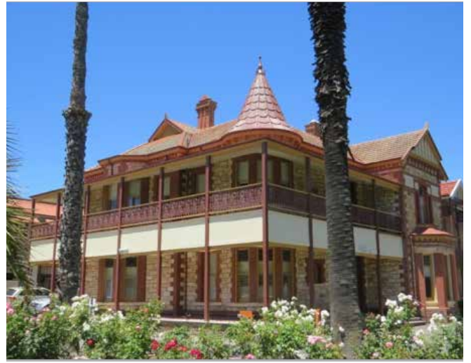
View to house, current
