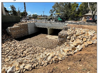
4 LBHC Daly Street Bridge
