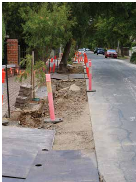
North Street, Frewville
