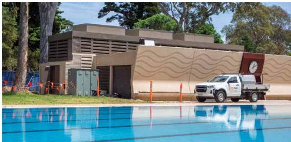
George Bolton Swimming Centre's new pool heater is powered through solar panels and will greatly decrease Council's emissions.
