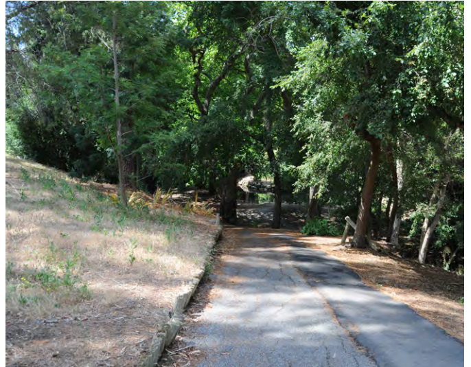
Hot mix pathways leading to pond area, looking east
