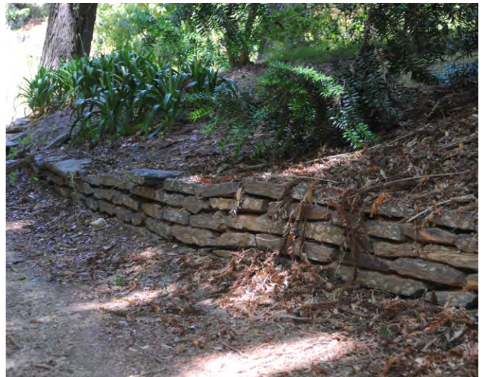
Dry stone retaining wall
