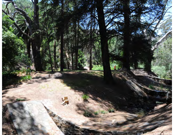
Drop structures within creek bed
