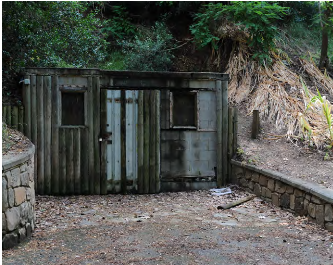
Garden shed and mortared stone retaining walls
